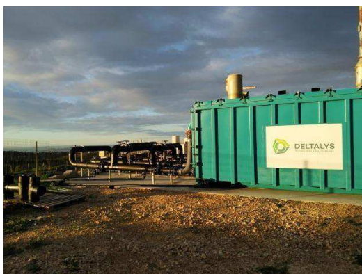
Photo 24 : Installation purification de l' H_2S
